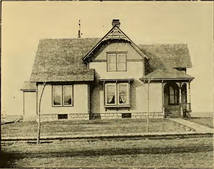
RESIDENCE OF S. H. KERR, ROLFE.
