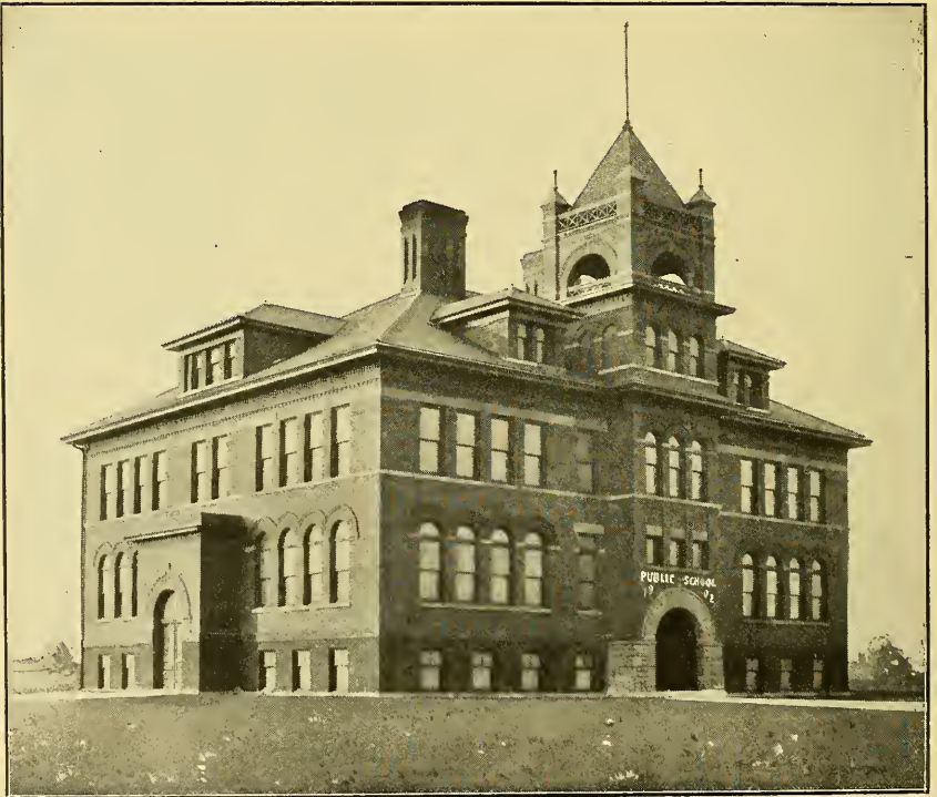
PUBLIC SCHOOL BUILDING, POCAHONTAS, 1902.
