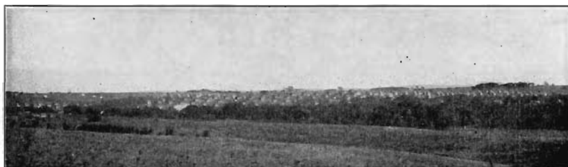
Figure 55. View of Buxton from the west.
