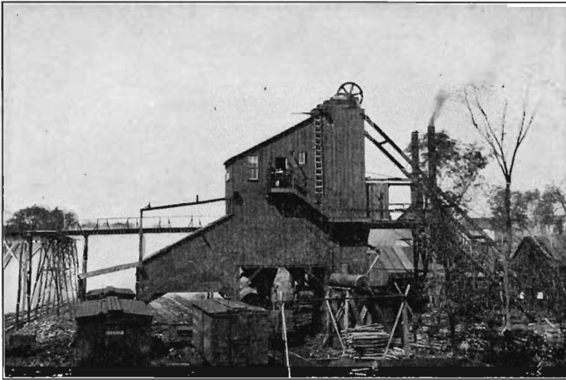
Figure 57. Tippel of shaft No. 2, Hocking Coal Company, Hocking.
